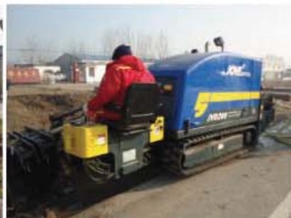
河北沧州施工现场 Jobsite in Cangzhou Hebei
