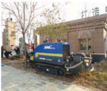
银川施工现场 Jobsite in Yinchuan
