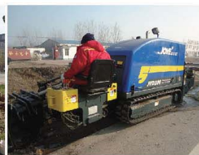
河北沧州施工现场 Jobsite in Cangzhou Hebei
