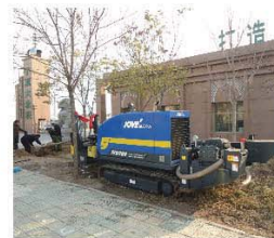
银川施工现场 Jobsite in Yinchuan
