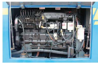
安装后的柴油机 After the installation of the diesel engine
